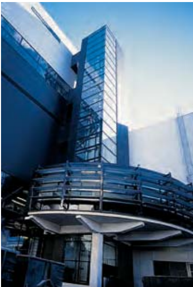
I/S Nordforbrænding in Hørsholm, Denmark, has installed a system to reduce the emission of NO x .
