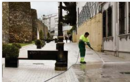
Furniture / Facade cleanig and repair
