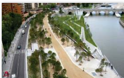
Irrigation and lighting
