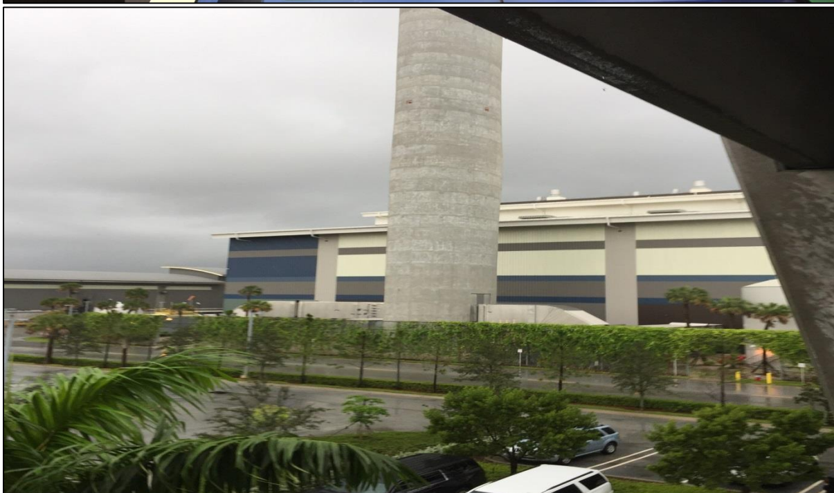
Photographs Solid Waste Authority of Palm Beach County Waste Facility
