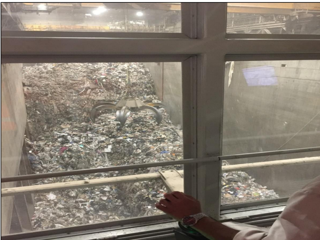
Photographs Corey Incineration Facility - London
