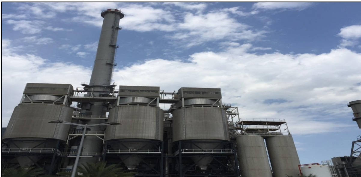
Photograph Ecoparc Facility in Barcelona
