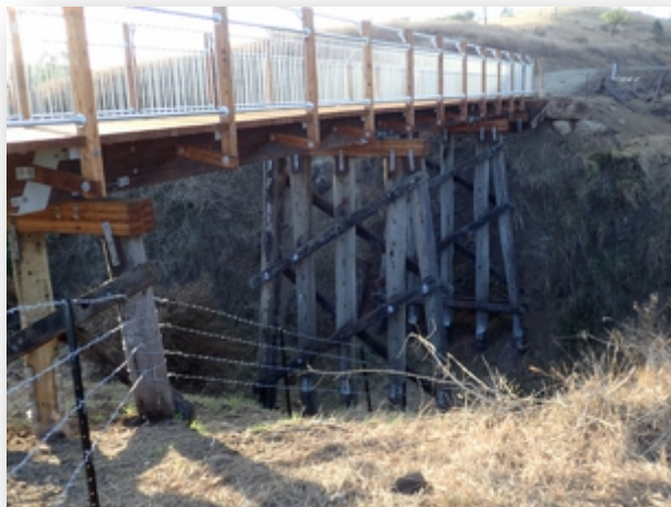
Repair work on the bridge over Jimmy’s Gully (on left) on the Brisbane Valley Rail Trail was complex and cost $11,000/lineal metre. The Tingoorra bridge on the Kingaroy Kilkivan Rail Trail (on right) was around $1,700 lineal metre for re-purposing.
