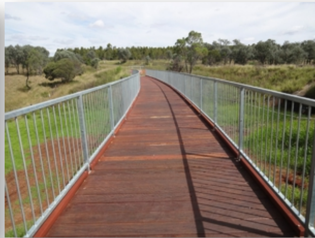
Repair work on the bridge over Jimmy’s Gully (on left) on the Brisbane Valley Rail Trail was complex and cost $11,000/lineal metre. The Tingoorra bridge on the Kingaroy Kilkivan Rail Trail (on right) was around $1,700 lineal metre for re-purposing.
