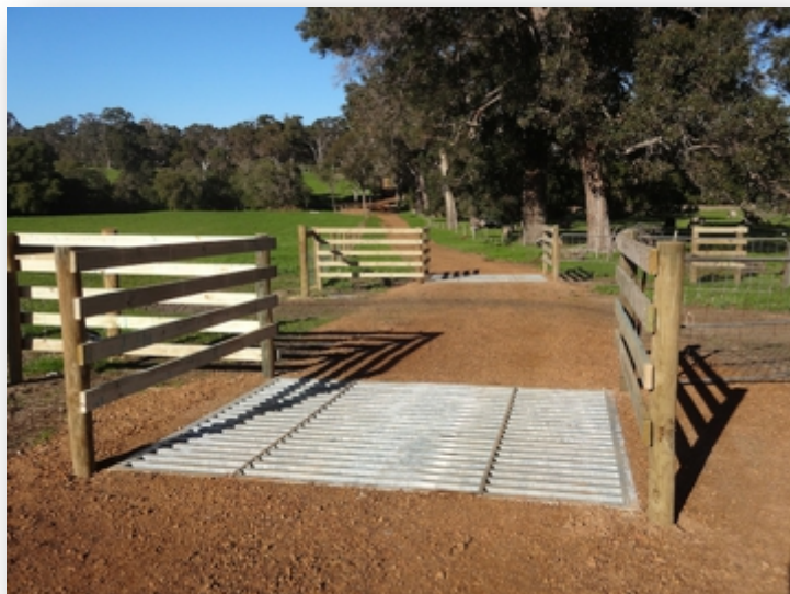
Stock grids along rail trails, such as this one on the rail trail south of Margaret River in WA, can allow stock crossings to be open 24/7 thereby enabling stock and machinery to cross the trail unimpeded.
