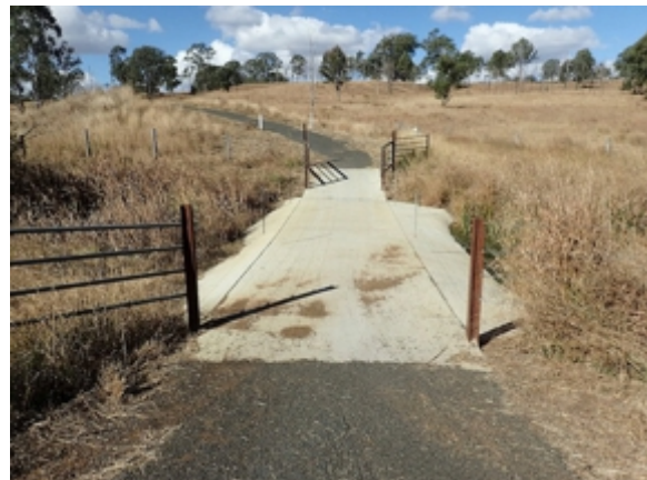
Above: A concrete floodway across a creek on the Kingaroy Kilkivan Rail Trail.
