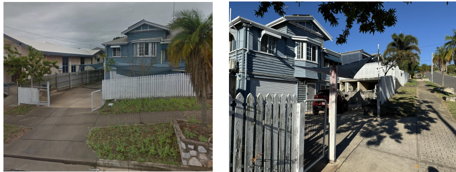
Existing double garage and entry at 200 Goondoon Street
