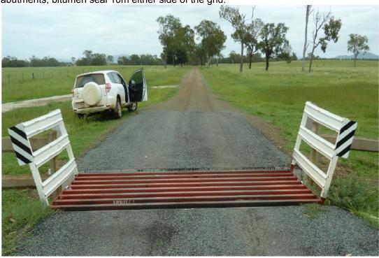
**Acceptable Condition** – This is a railway line grid with concrete abutments. RH wing is slightly bent however grid is structurally sound.
