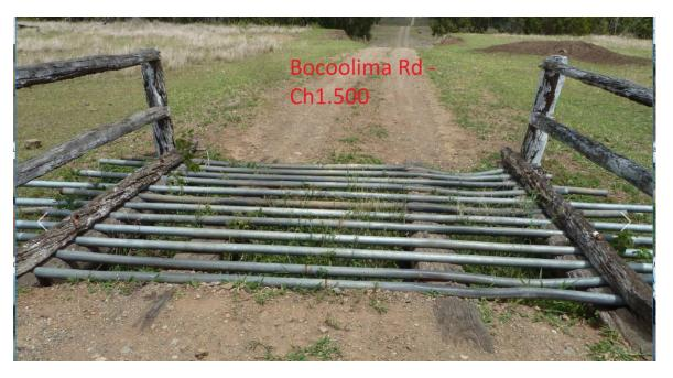
**Poor Condition** – This grid is of railway line construction with concrete abutments however the abutments are failing
