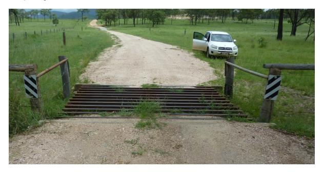
**Fair Condition** – Grid and abutments in sound condition however siderails and signs need to be fitted, once fitted this grid would be classed as acceptable condition.
