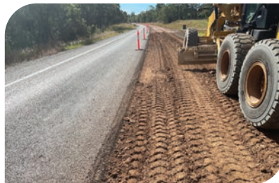
$2.3M Round Hill Road pavement renewal program
