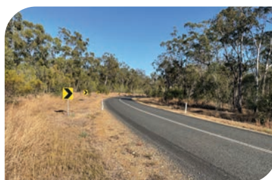
$1.1M Turkey Beach Road improvements
