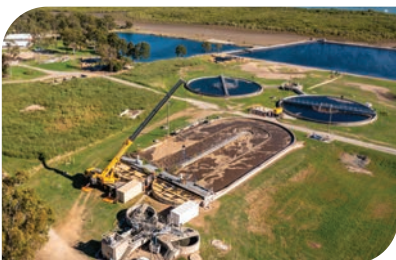
$2M Wastewater infrastructure upgrades
