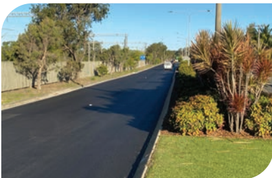
$2.5M Asphalt overlays and bitumen reseals
