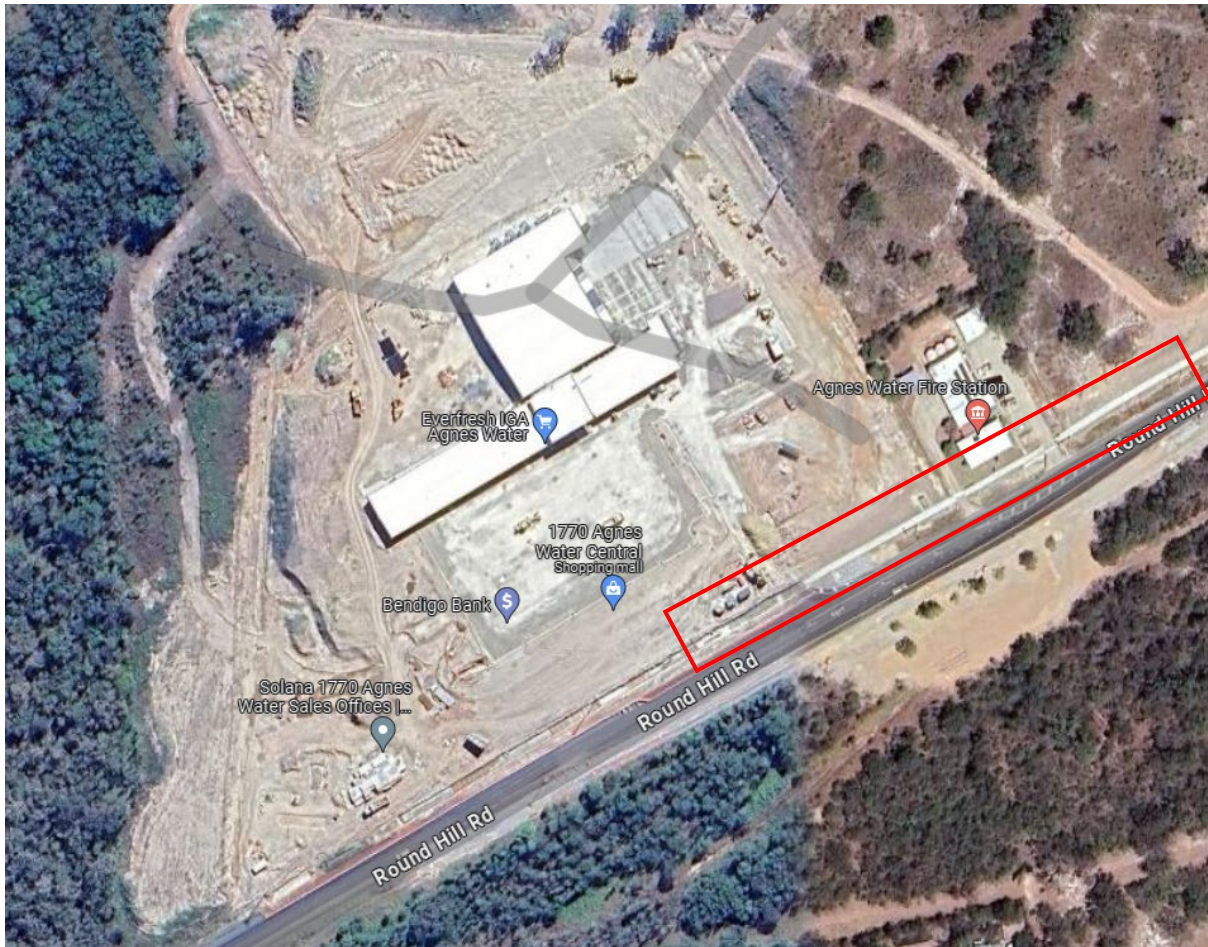
Figure 1: Recently constructed pedestrian footpath terminating at Lot 215 (Source Google Maps)
