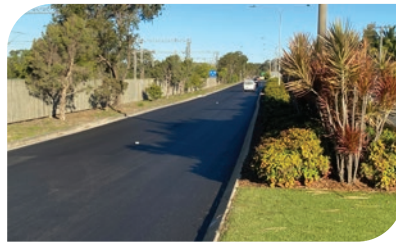
$2.1M Toolooa Street Gladstone Pavement Renewal
