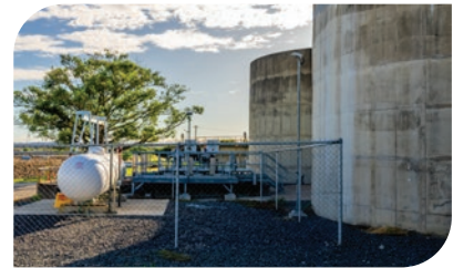
$2.2M Gladstone Waste Water Treatment Plant Upgrades
