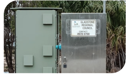
$3.5M Upgrade To Sewerage Pump Station A05
