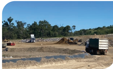
$2.4M Benaraby Landfill Cell Two Capping
