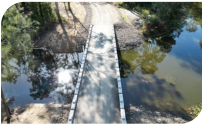
$2.5M Stockbridge Road Bridge Renewals
