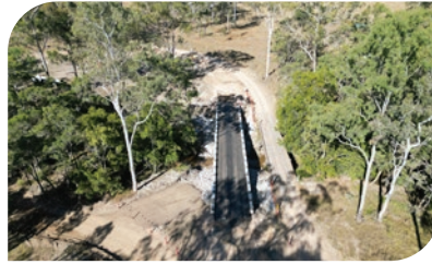
$3.6M Bindaree Road Bridge Upgrade
