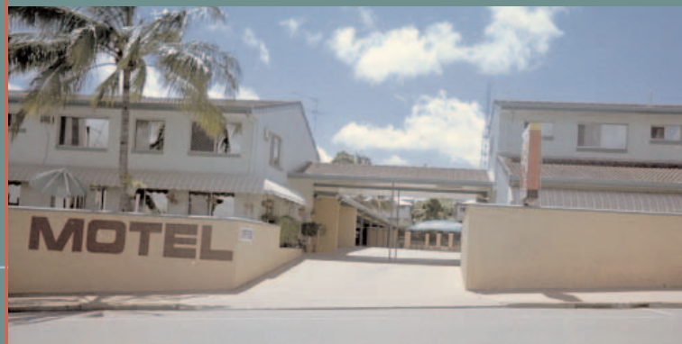
Blank walls pprovide inactive street frontage, reduce oppertunities for casual surveillance.
