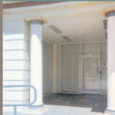
Doorways and building frontages set back impareing sightlines
