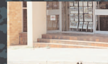
Many shops lack disabled access and do not provide active shop fronts
