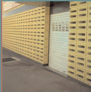
Shutters and building frontages do not provide active street frontage.
