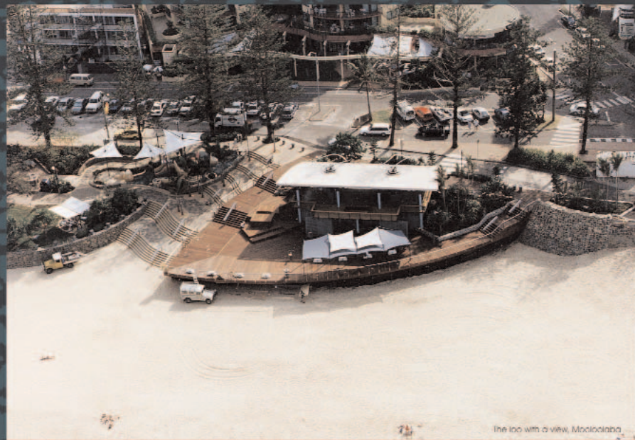
A landmark recreation space is required where Goodoon Street meets the waterfront.
