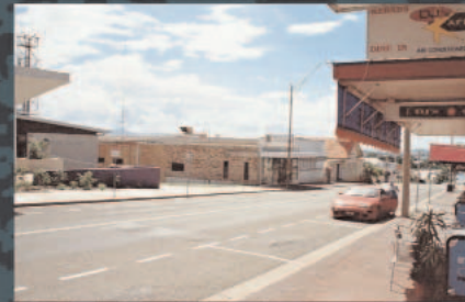
Blank walls surround the library
