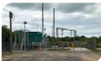
$1.2M upgrade to sewerage pump station A06
