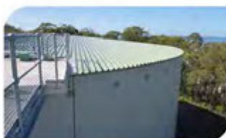
$1M Radar Hill Reservoir renewal
