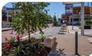
$1.4M Goondoon Street footpath
