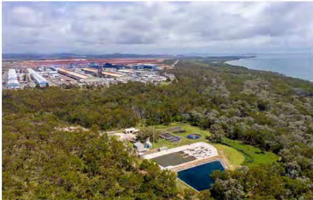
Boyne Island waste water treatment plant
