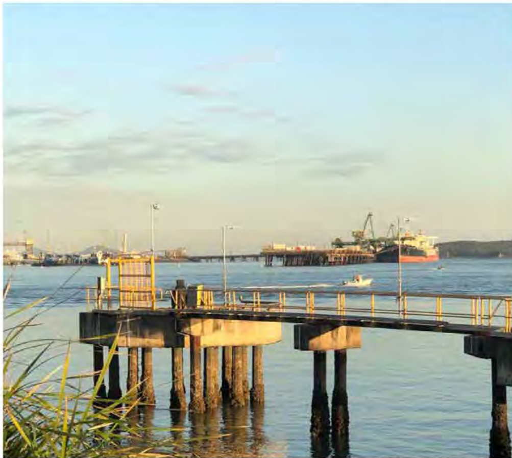
Looking towards the Port of Gladstone's RG Tanna Coal Terminal where four wharves are used to export coking coal to Japan, South Korea, Taiwan, India, Italy and France
