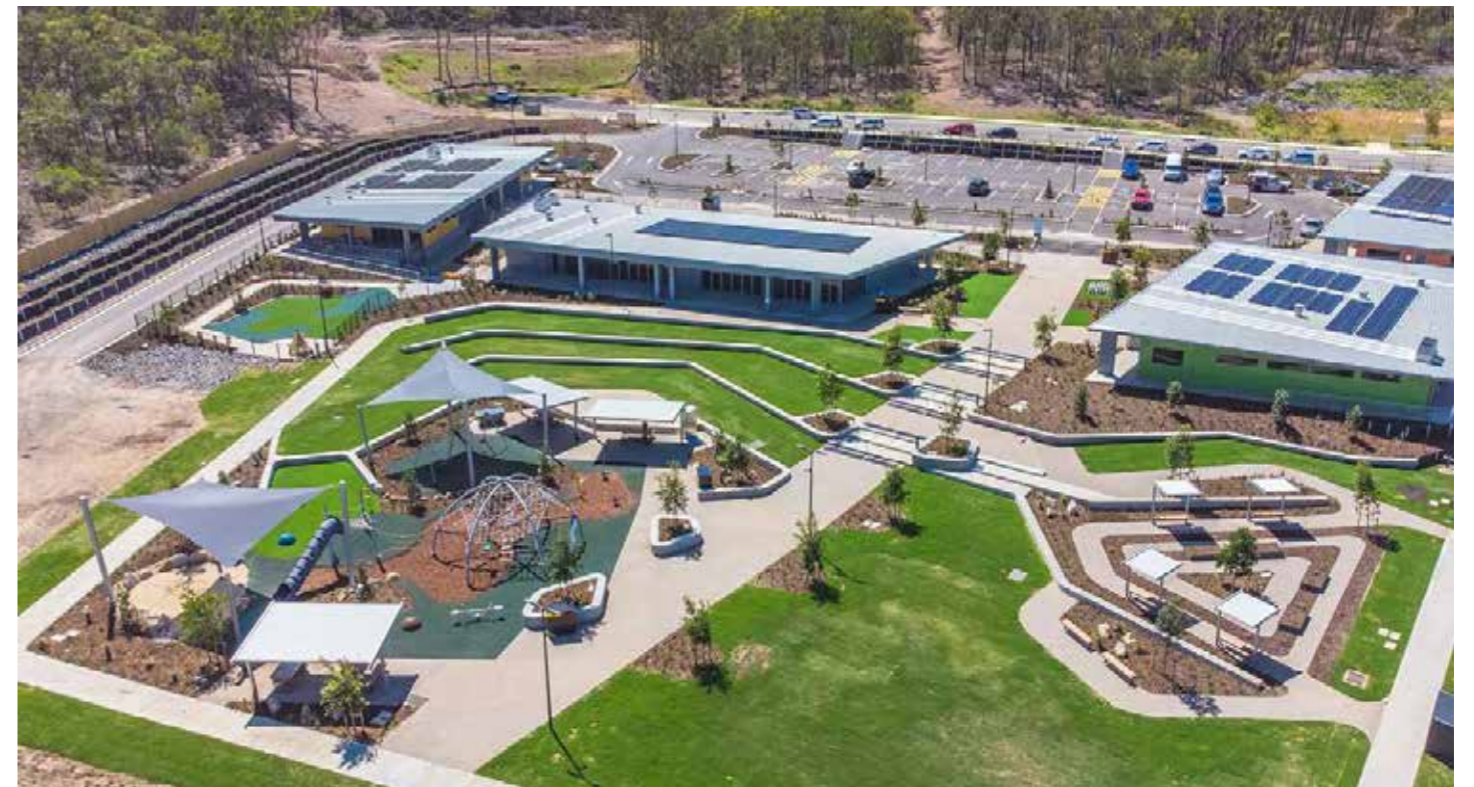
Figure 38: Philip Street Communities and Families Precinct (Source: https://paynters.com.au/project/philip-street-communities-and-families-precinct/ )
