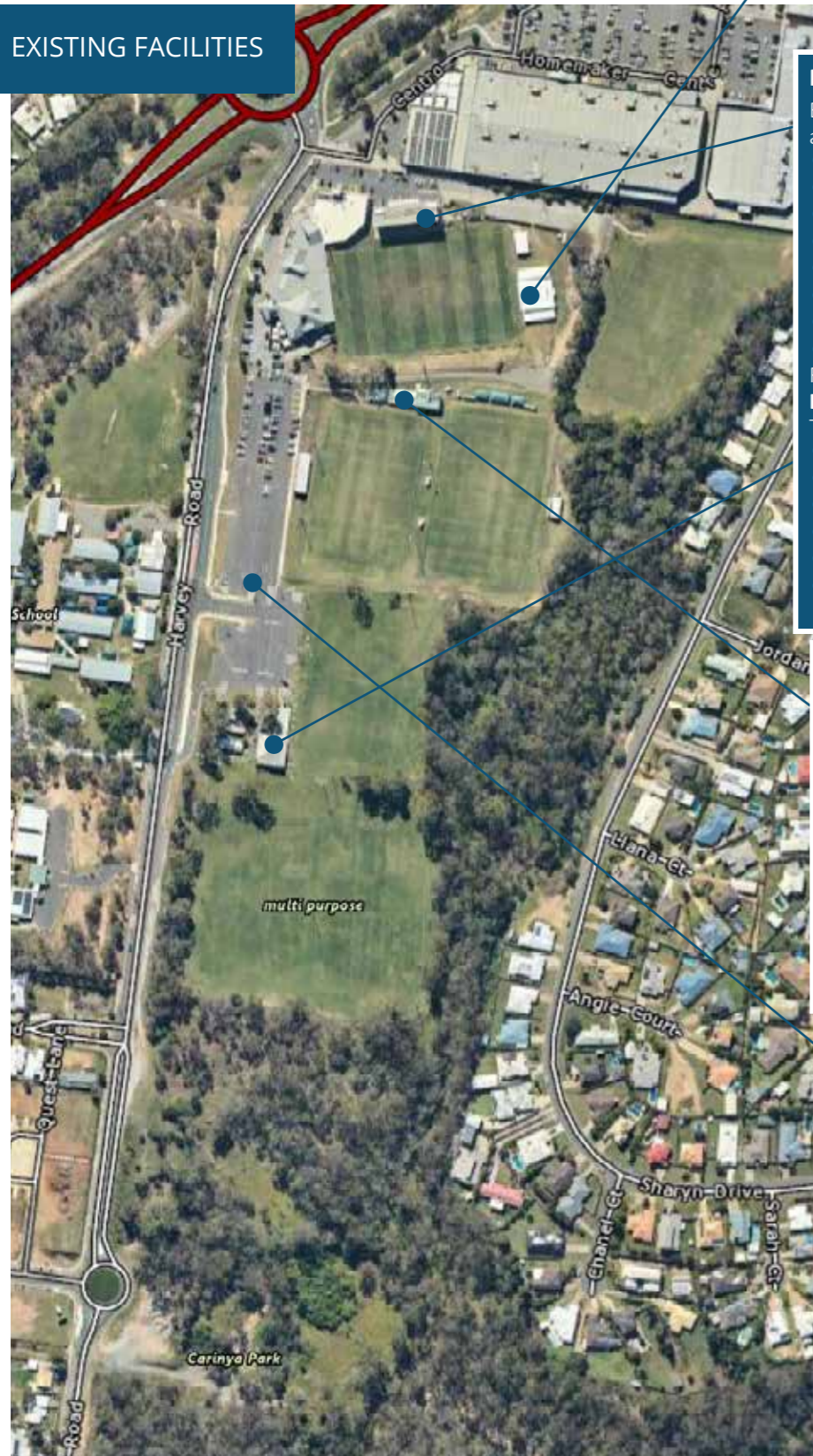
Figure 5: Existing facilities aerial
