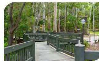
$1.4M Gladstone Tondoon Botanic Gardens external lighting upgrade
