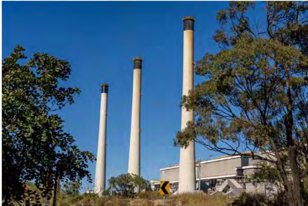
Gladstone's NRG Power Station began operating in 1976 and supplies electricity to aluminium producer, Boyne Smelters Ltd, under a long-term agreement
