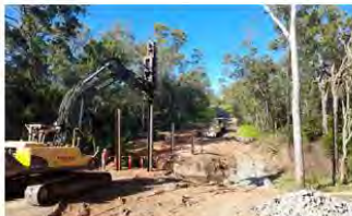
Bridge replacement John Clifford Way, Hobble Creek
