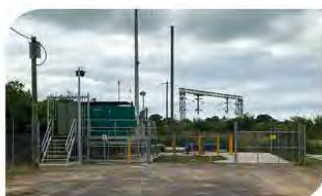
$1.2M upgrade to sewerage pump station A06
