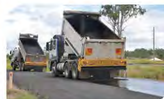
$1.5M asphalt overlays and bitumen reseals across the region
