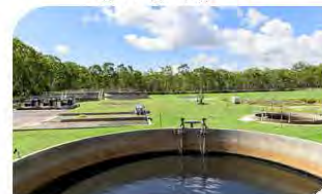
$1.8M relining South Trees treatment ponds
