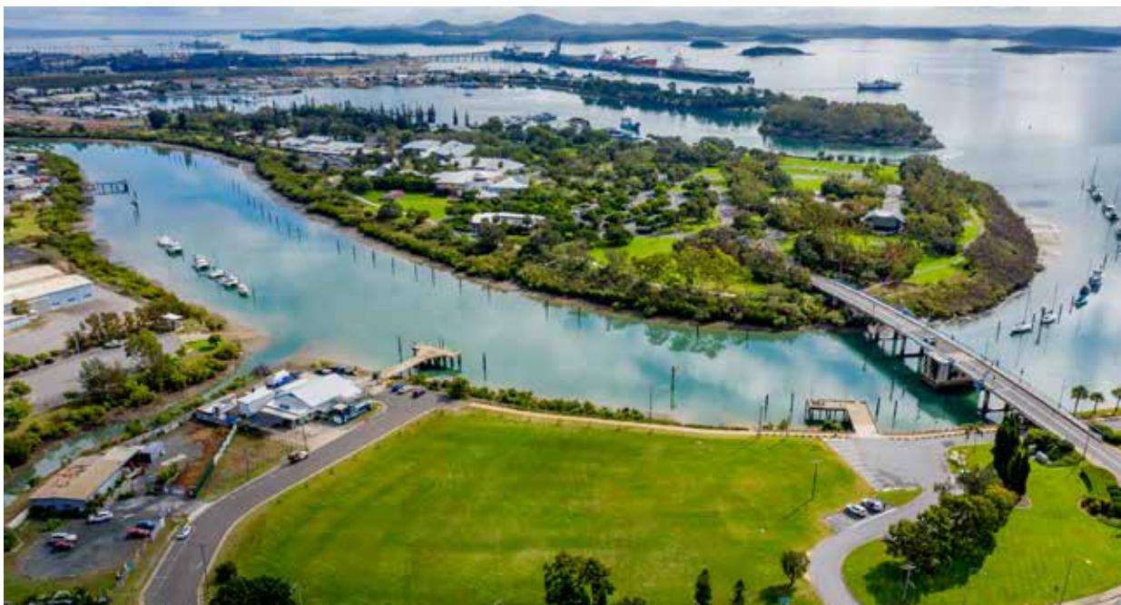
The Gladstone Marina bridge (foreground) links the central business district to the marina parklands and RG Tanna Coal Terminal
