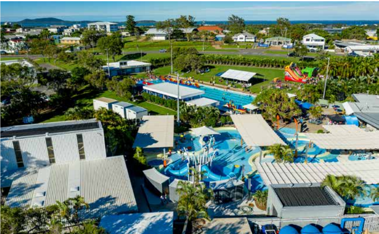
The Gladstone Aquatic Centre is in the Green Belt that runs through the centre of the city, adjacent to the Central Business District
