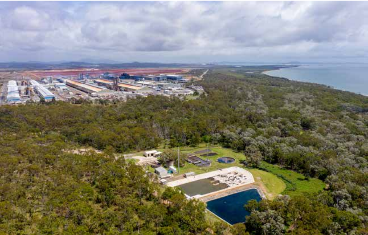
Boyne Island waste water treatment plant
