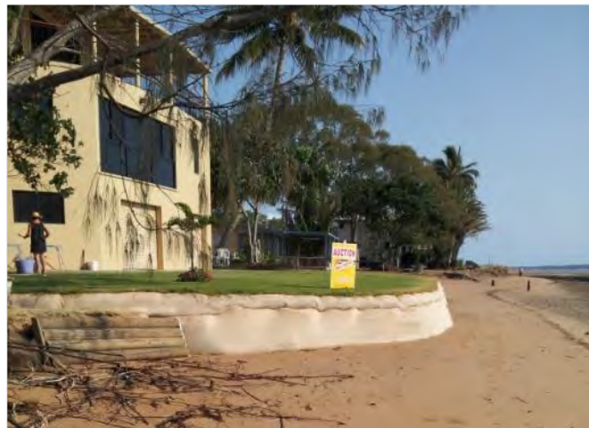
Plate 7 - Retaining wall constructed by resident on public land
