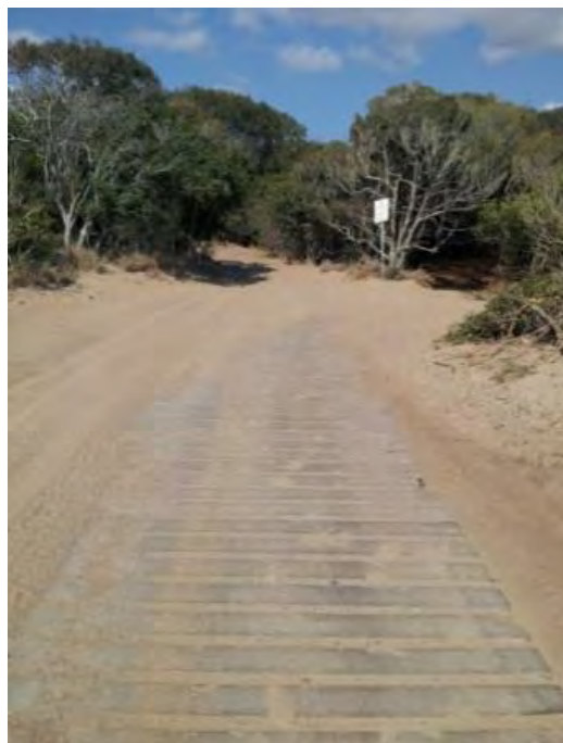
Plate 2 - View of access point to Lilley's Beach comprising of board and chain path
