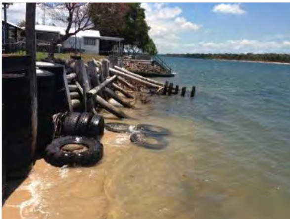
Plate 17 - Groynes made from tyres installed by residents on mainland side of Colosseum inlet
