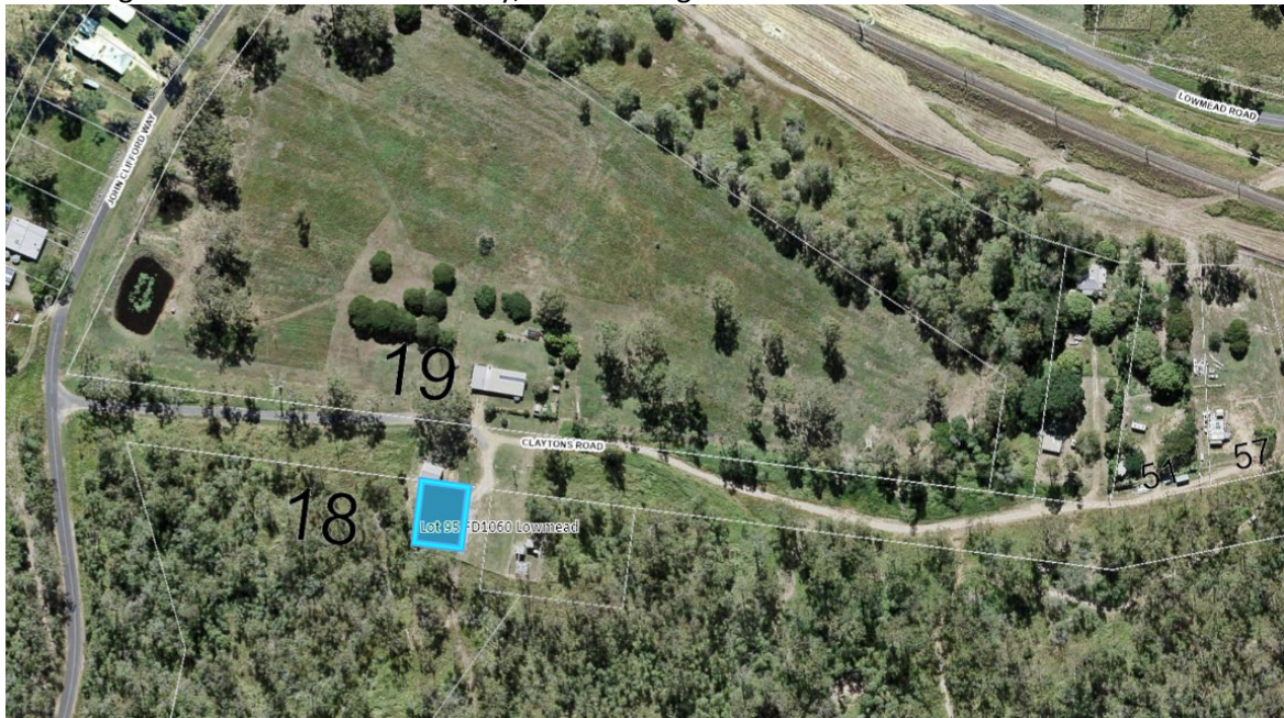
Lowmead Rural Fire Brigade – Claytons Road note - slight error in Geocortex overlay, RFB building is located on Lot 95
