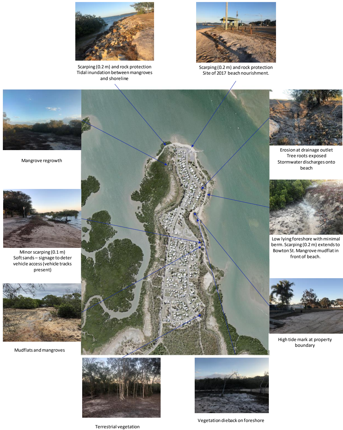
Figure 41. Summary of key site inspection observations
