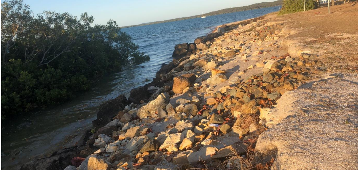
Figure 19. Northern point shoreline – informal rock protection at far western side of the point
