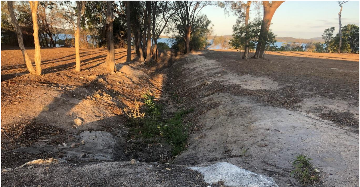
Figure 24. Eastern shoreline - stormwater drainage at the northern section of beach at Bell Street
