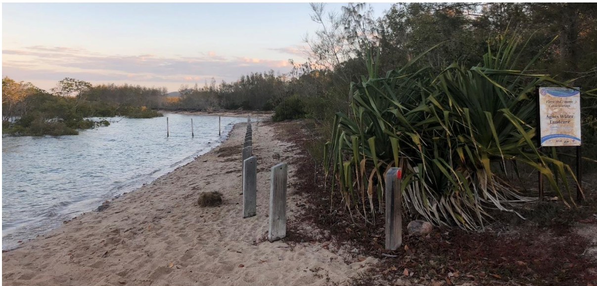
Figure 25. Eastern shoreline – timber bollards
