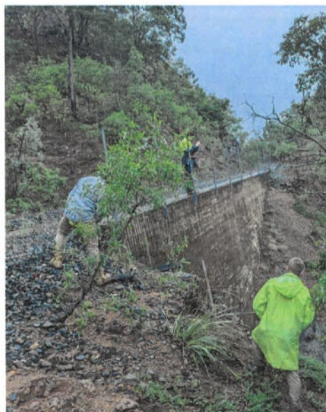
Typical steep embankments around existing retaining structure
