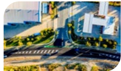
$1.9M Blain Drive, Gladstone - Pavement Renewal
