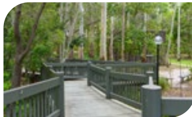
$1.7M Gladstone Tondoon Botanic Gardens External Lighting Upgrade
