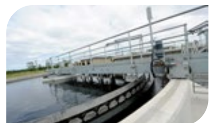
$2.3M Boyne Island Waste Water Treatment Plant - Belt Press and Shed
