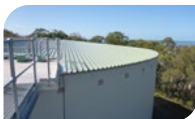
$2.2M Ferris Hill Reservoir Renewal
