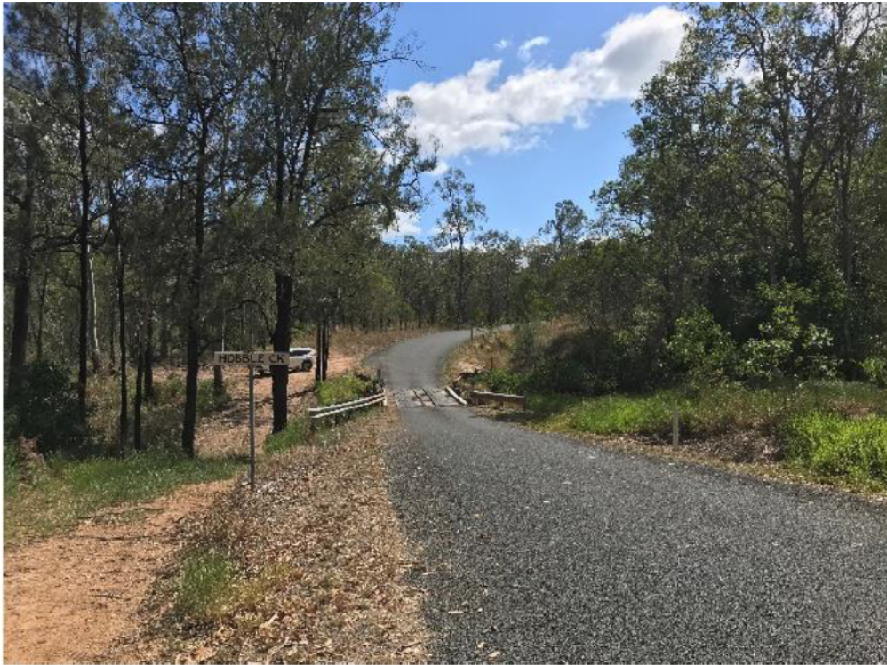
Figure 1 – Bridge over Hobble Creek on John Clifford Way, Lowmead
