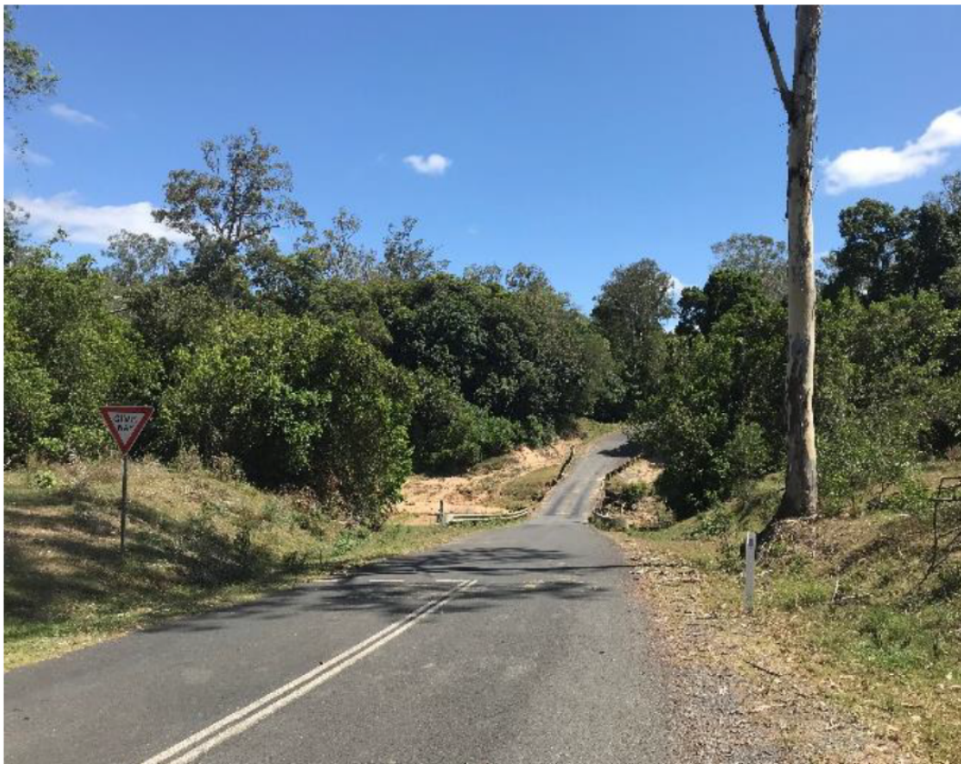
Figure 2 – Bridge over Baffle Creek on Gorge Road, Lowmead.
