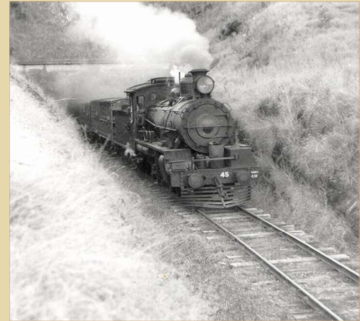
Train leaving Yimbun Tunnel. Photo courtesy of Brisbane Valley Heritage Trails.
