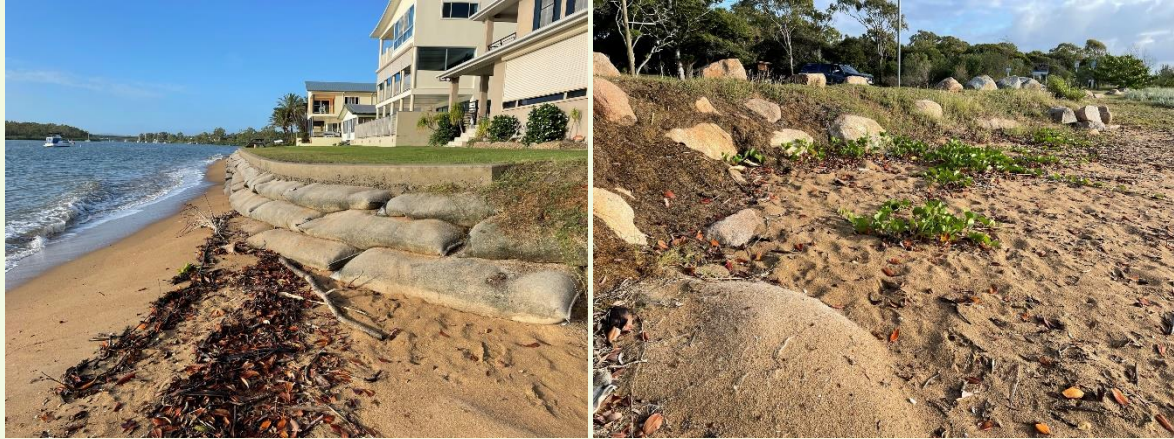
Figure 25. Existing conditions at Lilley's Beach entrance.
