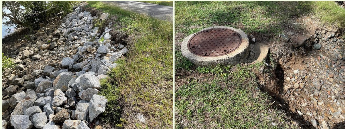
Figure 30. Existing conditions at Turtle Way.
