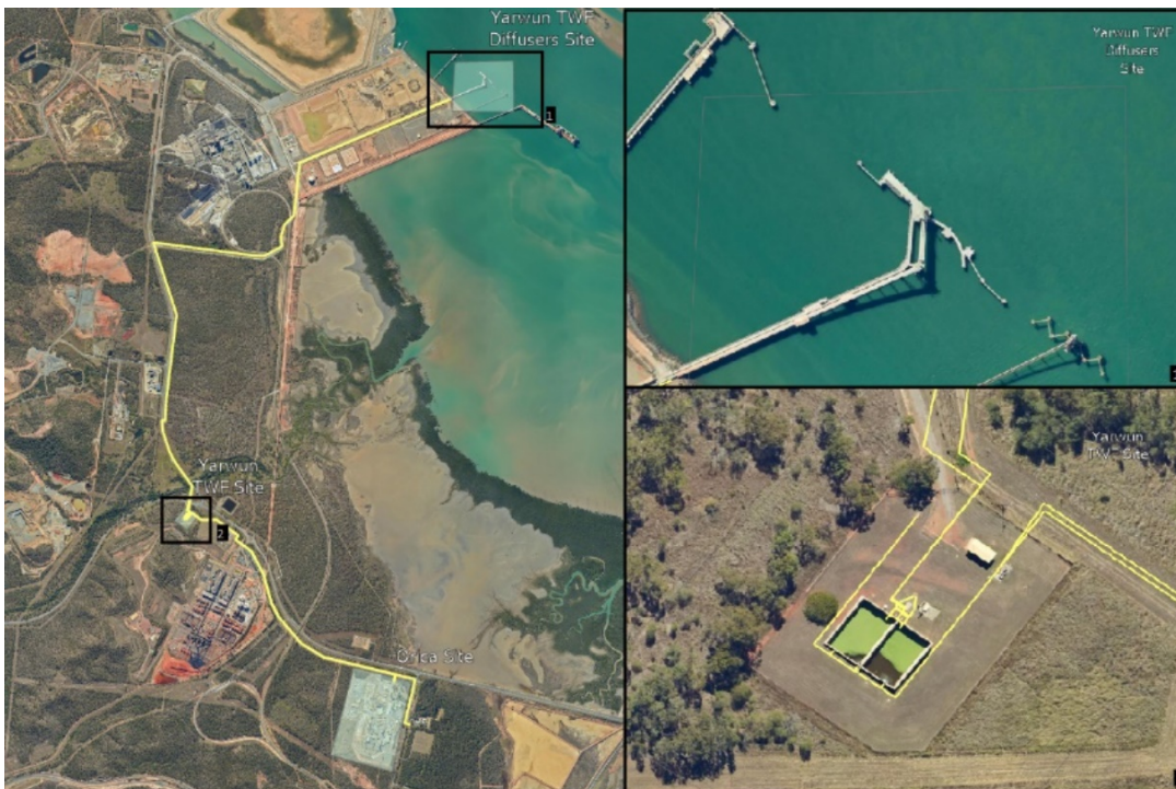
Figure 1 - Yarwun Tradewaste Facility
